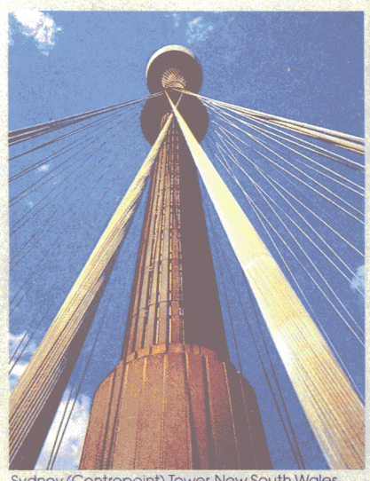
Sydney (Centrepont) Tower, New South Wales
